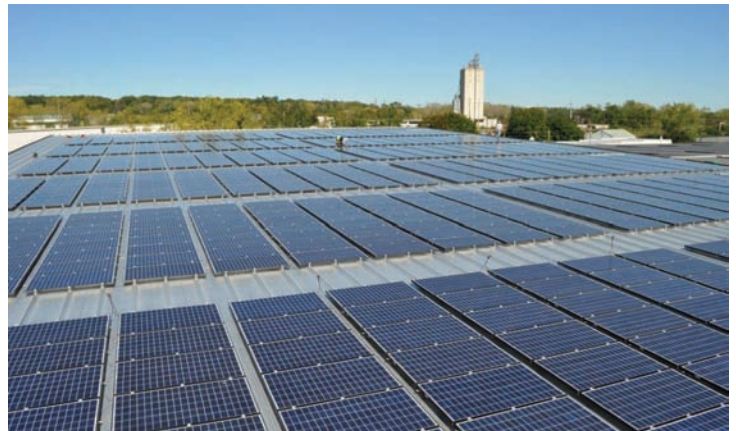
Solar panels installed on the Henry Molded Products warehouse roof in Lebanon, PA.
